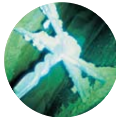
Steel wall-tie inside brick cavity wall
