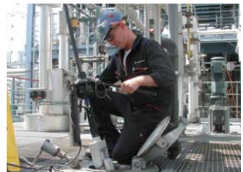
Tank and vessel inspection
